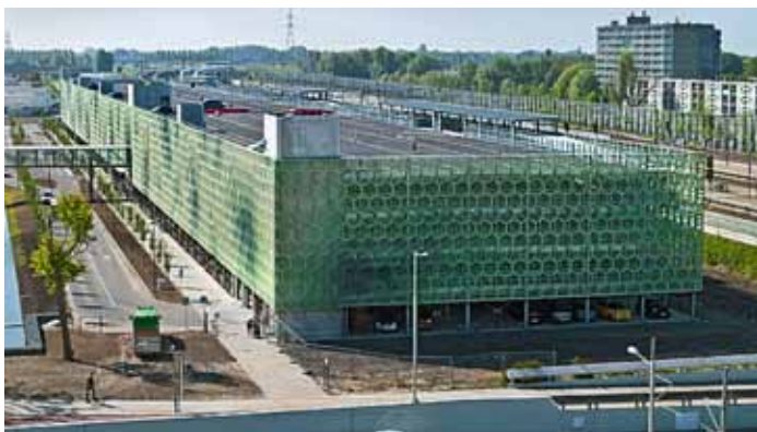
3.14 Medimall car park in Rotterdam (Netherlands), in which the fire engineering method considering physical, local fires was applied.
