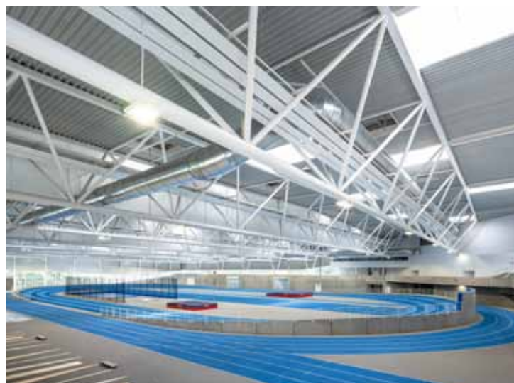
3.1 With fire safety engineering attractive (fire) safe buildings can be achieved, like this sports hall with an indoor athletics track and a free span of 80 m in Louvain-la-Neuve (Belgium).
